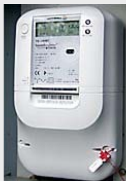
Box with GPRS-Transmitter and PLC System
